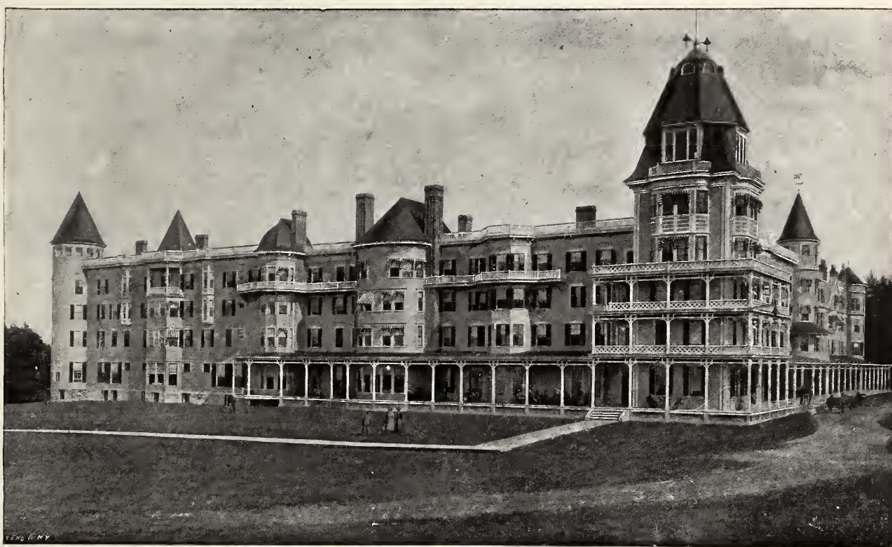
NORTHWEST FRONT POLAND SPRING HOUSE
